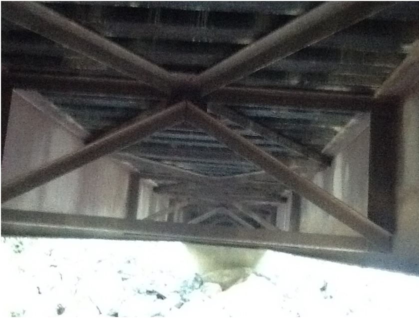
Underside of bridge
