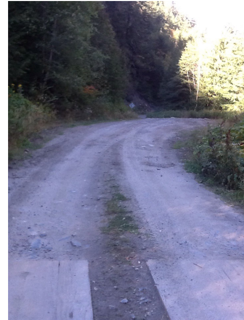
Left approach facing away from structure
