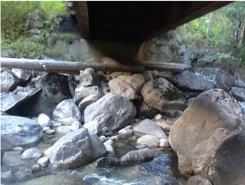
Left Bank Abutment when facing downstream
