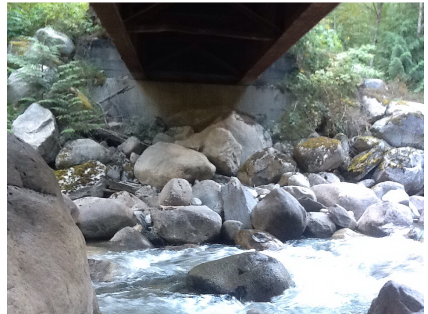
Right Bank Abutment when facing downstream
