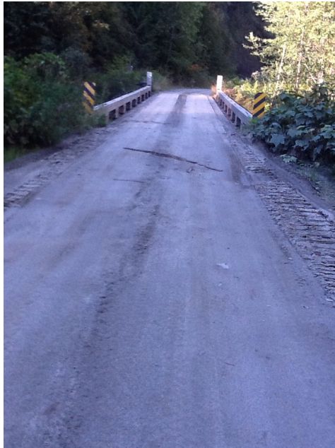
Right approach facing structure
